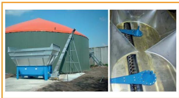
Figure 3.6: Receiving vessel with loosener [Konrad Pumpe GmbH]
