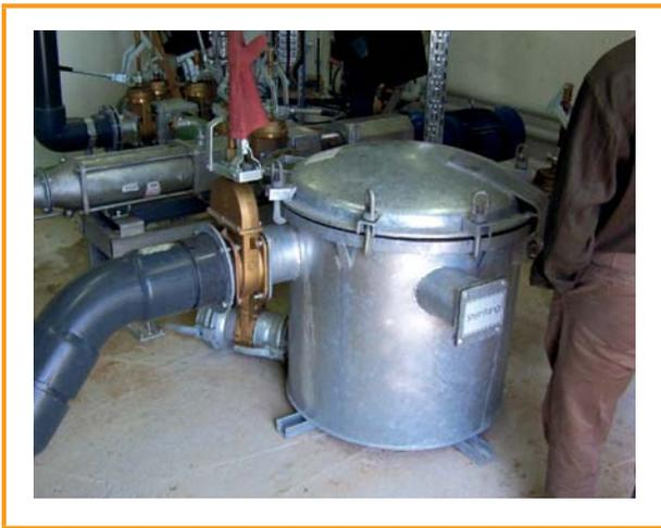
Figure 3.5: In-pipe separator for dense materials [DBFZ]
