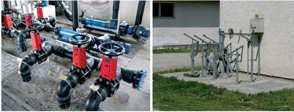
Figure 3.20: Pipes, valves and fittings in a pump station, shut-off gate valves [DBFZ]
