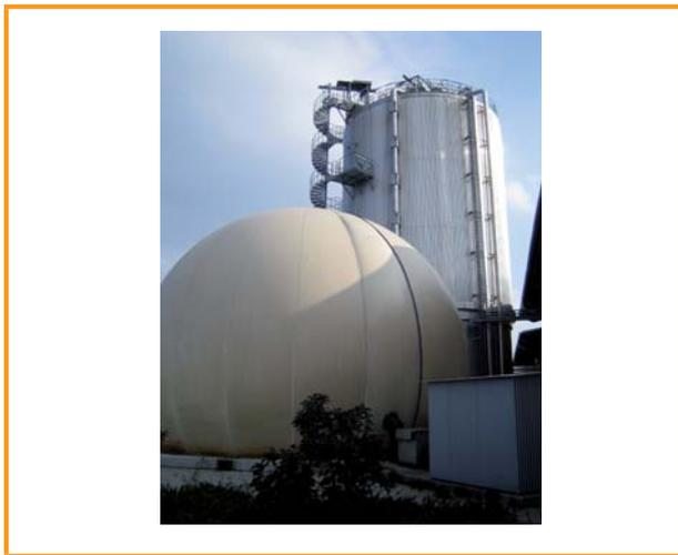
Figure 3.40: Example of a freestanding plastic-sheeting storage tank with two thicknesses of plastic sheeting [Schüsseler, FNR]
