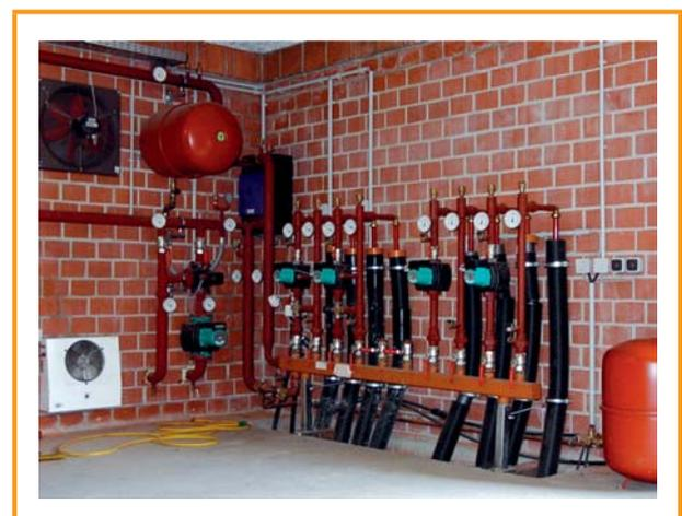
Figure 6.7: Heat distributor [MT-Energie GmbH]
