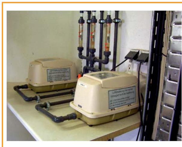
Figure 6.1: Gas control system for injecting air into the digester gas space [DBFZ]
