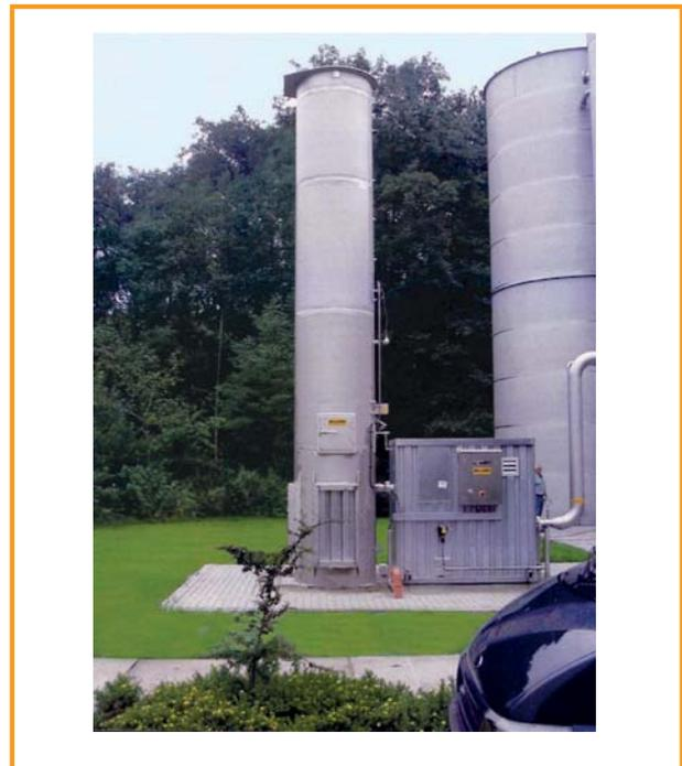
Figure 3.41: Emergency flare of a biogas plant [Haase Umwelttechnik AG]
