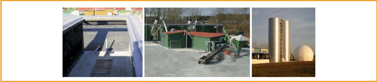
Figure 3.28: Examples of special constructions in dry digestion; sequential batch reactor (left), stirred-tank box digester (centre), methanisation stage of the dry/wet digestion process and external gas storage tank (right) [ATB Potsdam (left), Mineralit GmbH (centre), GICON GmbH (right)]
