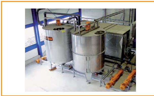
Figure 3.10: Hygienisation with recooling [TEWE Elektronik GmbH & Co. KG]
