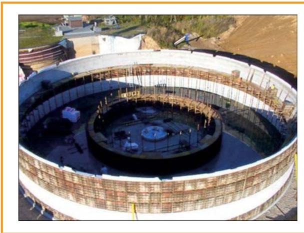
Figure 3.29: A concrete digester under construction [Johann Wolf GmbH & Co Systembau KG]
