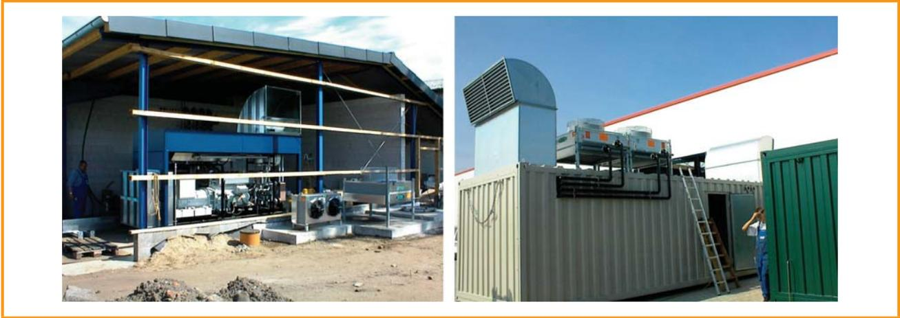
Figure 6.9: Installation of a CHP unit inside a building and in a CHP container [Seva Energie AG]
