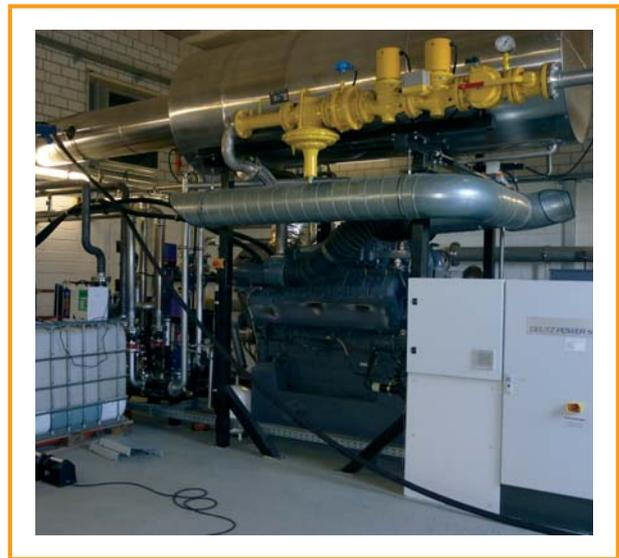
Figure 6.8: CHP unit with gas control train [DBFZ]
