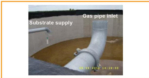
Figure 3.36: Provisions to prevent disruption of gas extraction; gas pipe inlet with intake opening upward (substrate feed inlet is to the left) [DBFZ]
