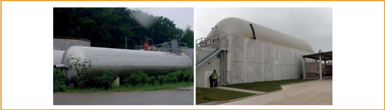
Figure 3.25: Plug-flow reactors; field examples, cylindrical (left), box section, with overhead gas reservoir (right) [Novatech GmbH (left), DBFZ (right)]
