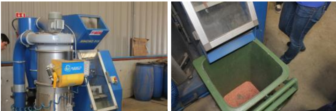
Figure 107 – Visit to the solid waste treatment and upgrading integrated center of Valnor
