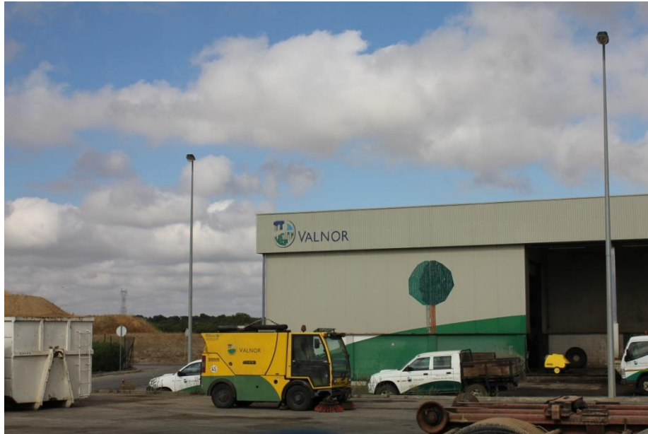
Figure 10 – Visit to the solid waste treatment and upgrading integrated center
