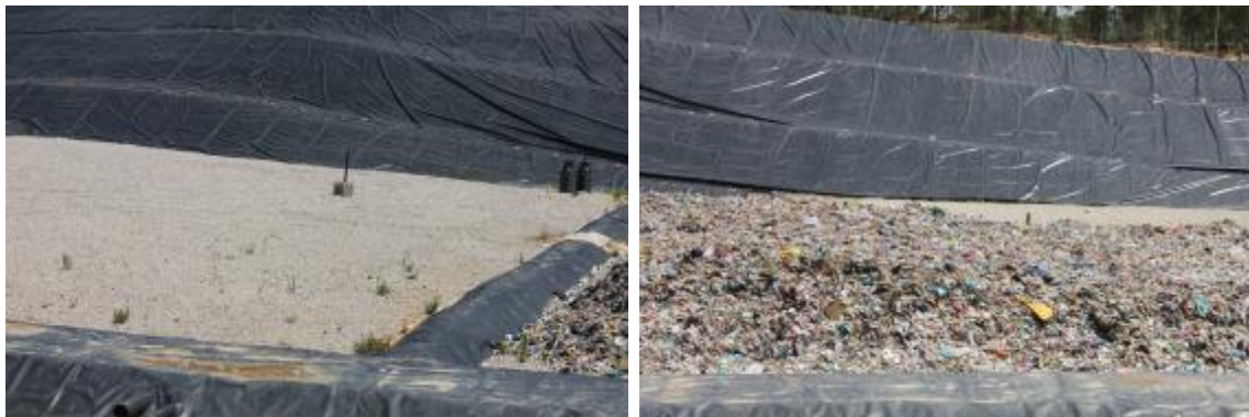
Figure 147 – Visit the landfill in operation with biogas capture of Valorlis
