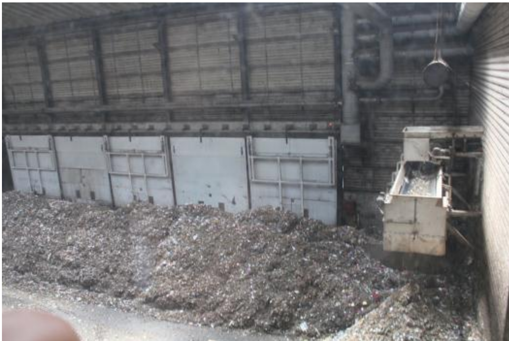
Figure 63 – Visit to the solid waste treatment and upgrading integrated center
