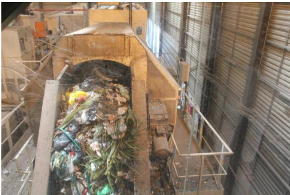
Figure 11 – Visit to the solid waste treatment and upgrading integrated center
