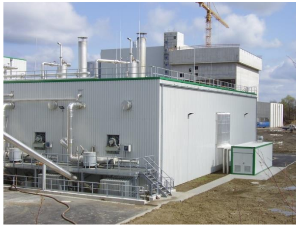
Figure 10: Biogas/biomethane plant Rostock, Germany (Source: EVG Entsorgungs-und Verwertungsgesellschaft mbH Rostock)
