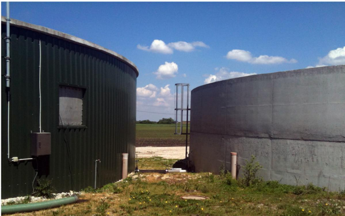
Figure 14: Digester and open lagoon for digestate
