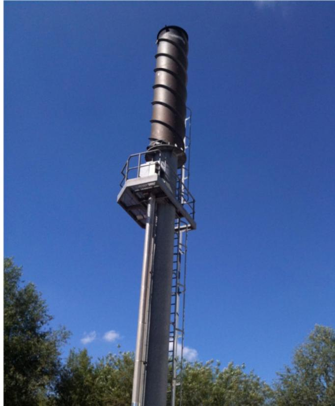
Figure 9: Biogas flare
