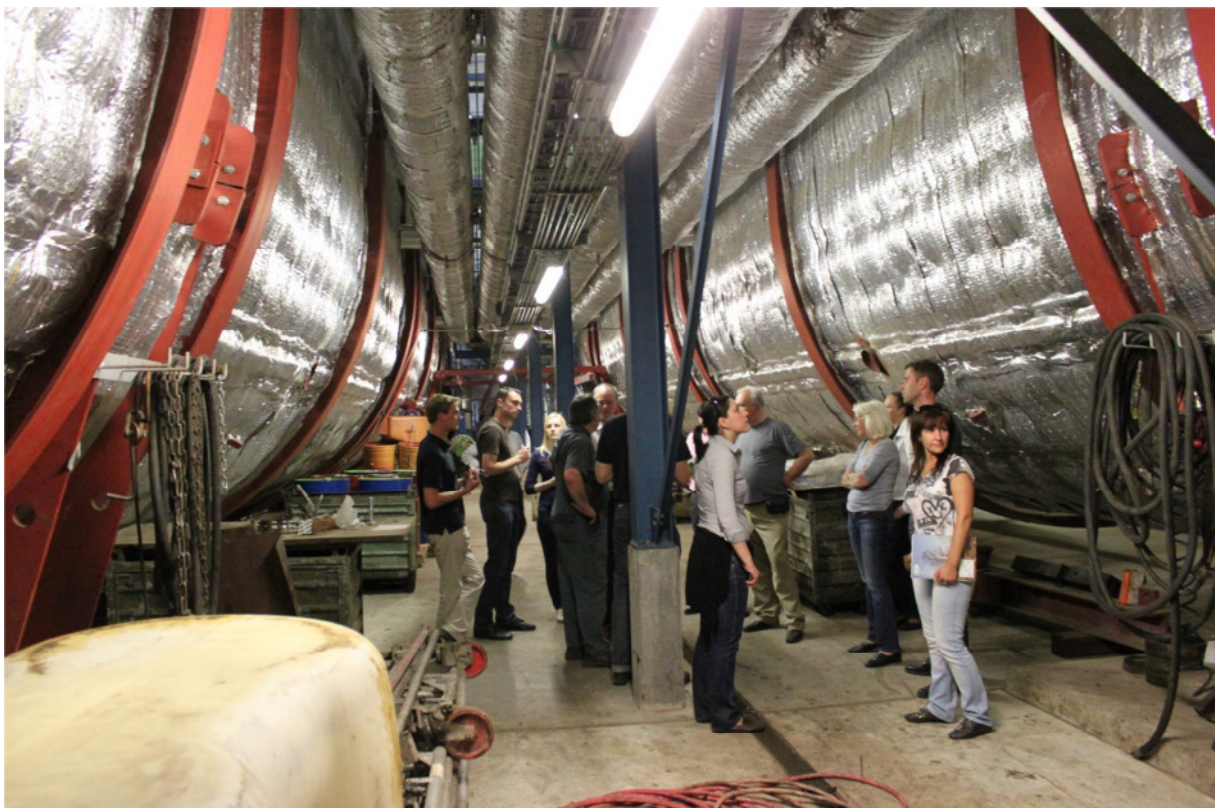
Figure 15: Digesters of the biogas plant for organic household waste of Wurzer Umwelt
