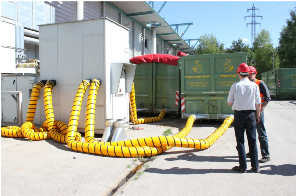
Figure 6: Heat of the CHP plant is used for woodchip drying at the Gansner biogas plant
