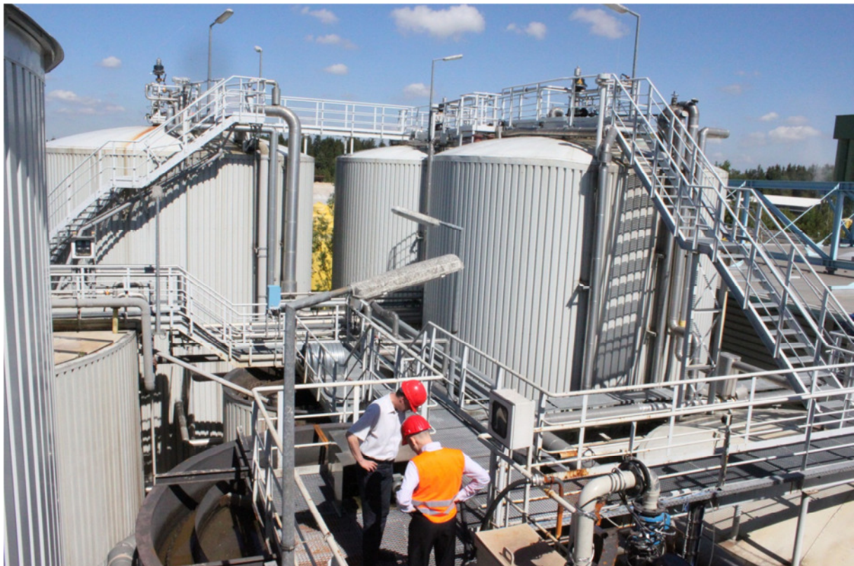
Figure 7: Digesters of the Gansner biogas plant
