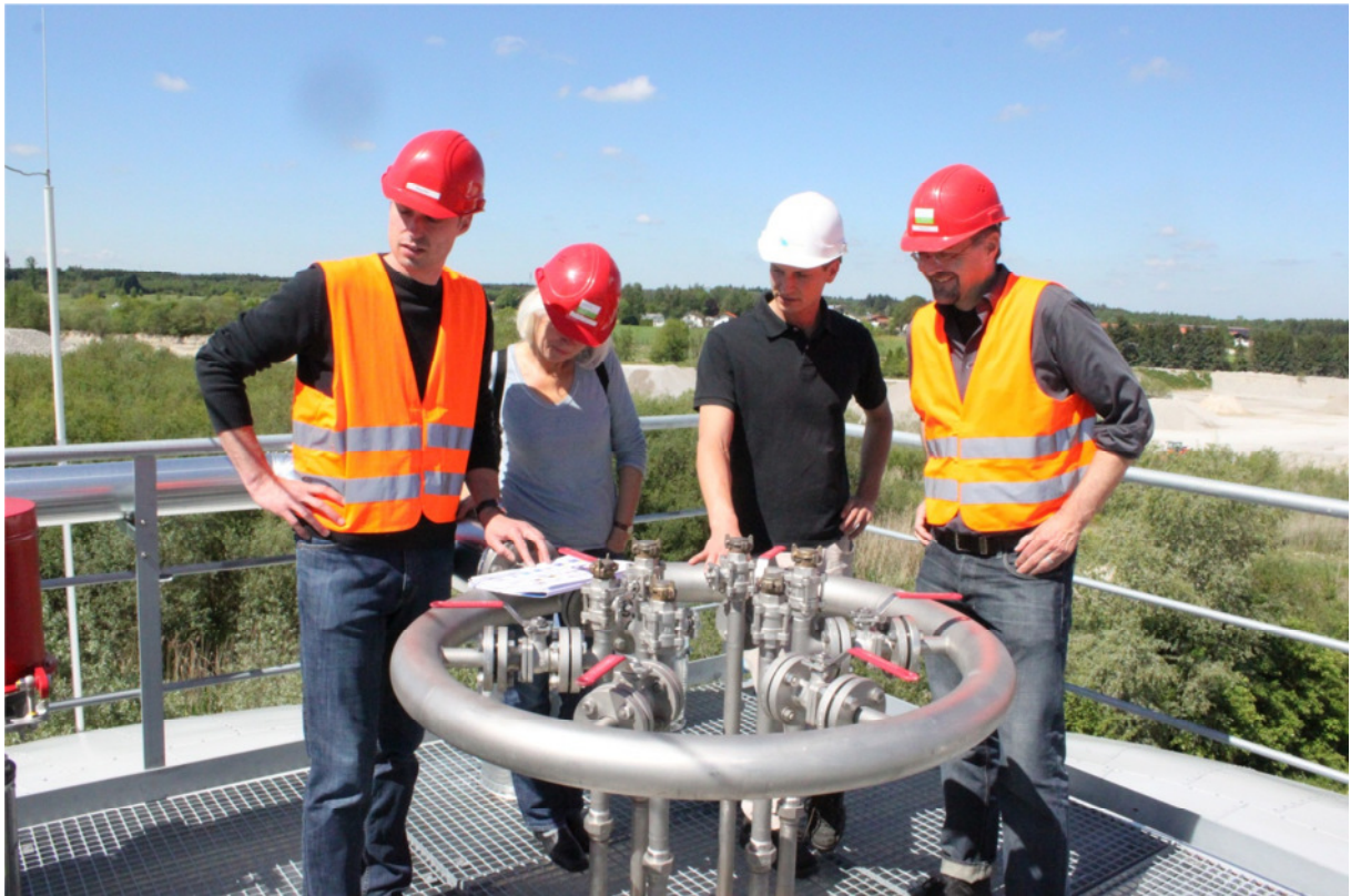
Figure 8: At the top of the Ganser biogas plant
