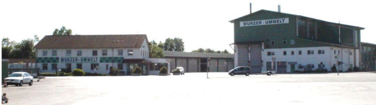
Figure 13: Facilities of Wurzer Umwelt
