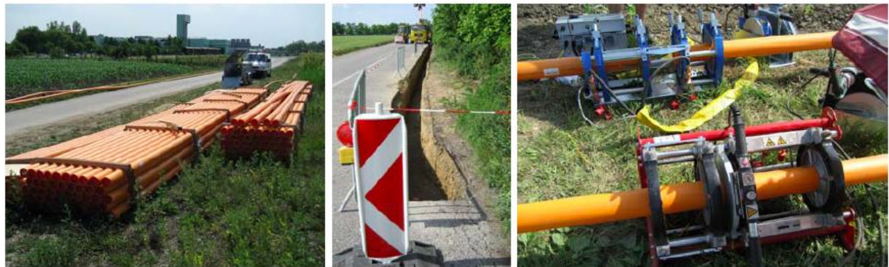
Figure 10: Biomethane pipeline in Bruck/Leitha, Austria during construction; pipe connection by welding (right); Source: Vienna University of Technology
