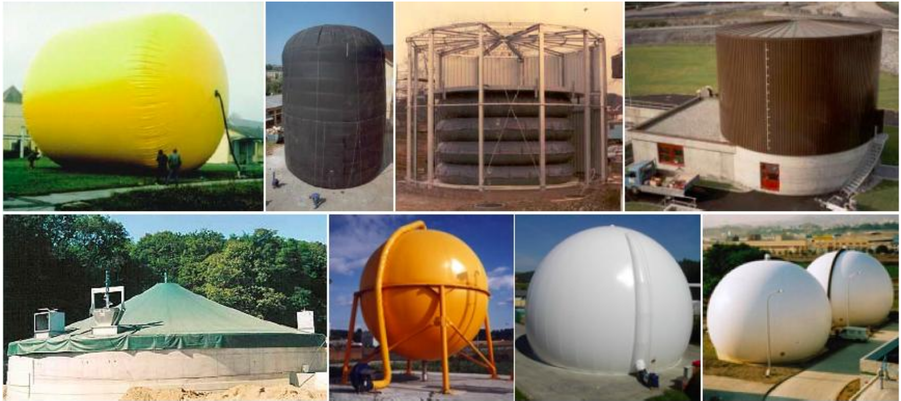
Figure 4: Low pressure gas storage systems: balloon type gas storage (upper row left); cushion type gas storage (upper row right); membrane roof gas storage on fermenter top (lower row left); external double membrane storage system (lower row right); Sources: Sattler AG and Panaqua AG
