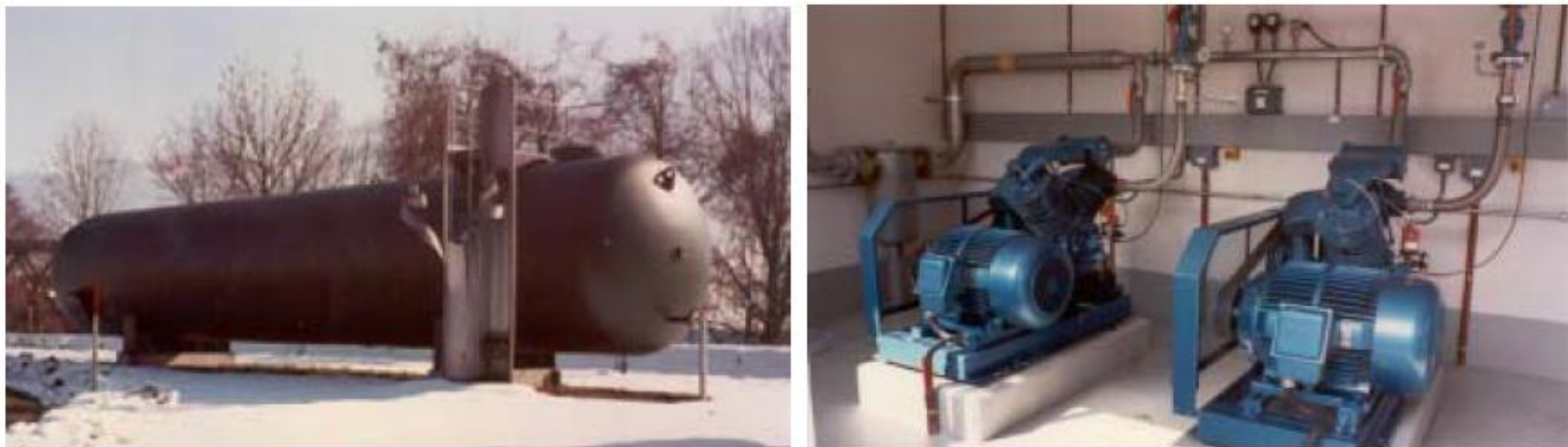
Figure 5: Raw biogas storage systems for elevated pressure: gas storage tank (left); compression and expansion unit (right); Source: Panaqua AG
