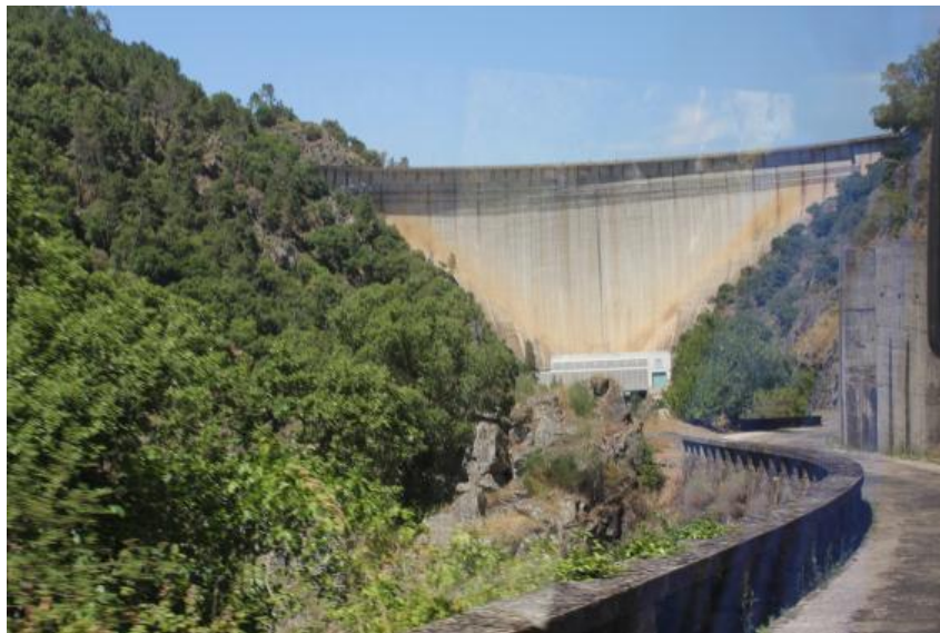
Figure 37 Visit to Hydro Central Production of Cabril
