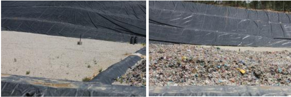
Figure 32 Visit the landfill in operation with biogas capture of Valorlis. Landfill cells
