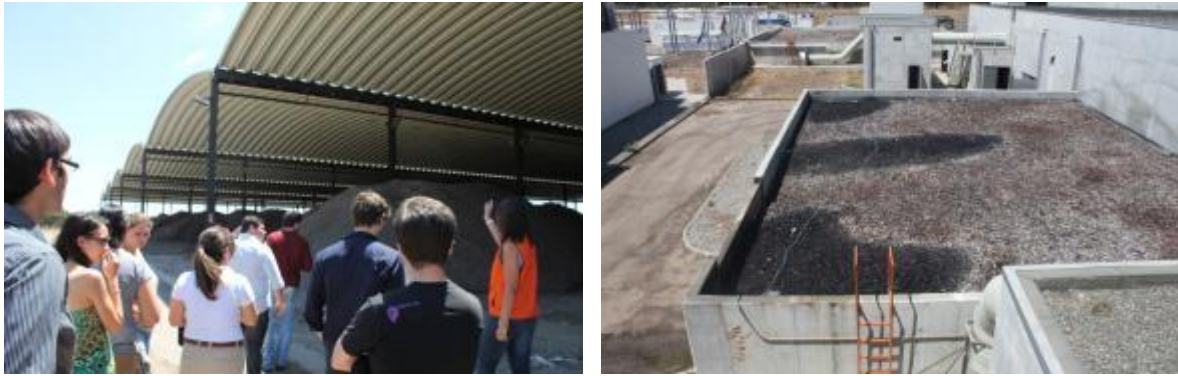
Figure 21 Visit to the solid waste treatment and upgrading integrated center of Valnor. Left the compound after anaerobic digestion and right biofilters for odors removing
