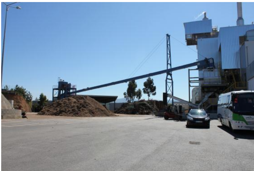
Figure 35 Visit to Biomass Central Palser facilities
