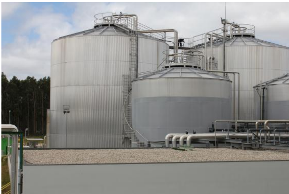
Figure 29 Visit to the the solid waste treatment and upgrading integrated center of Valorlis. Digestors
