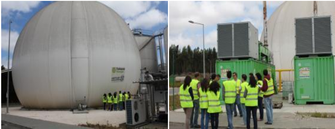
Figure 30 Visit to the solid waste treatment and upgrading integrated center of Valoris. Gasometer at the left and at right motor generators
