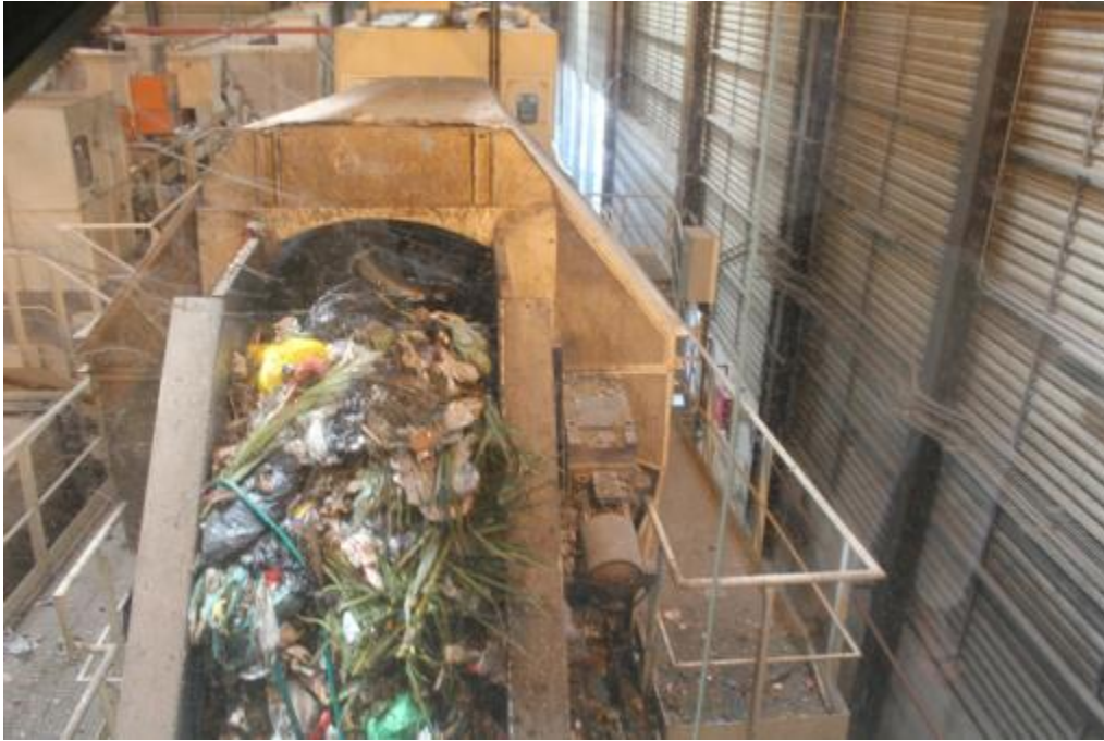
Figure 17 Visit to the solid waste treatment and upgrading integrated center. Entrance of the waste for the automatic separation line
