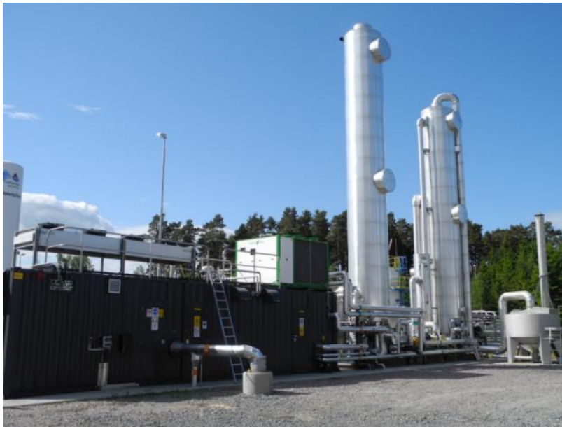
Picture 16: Water scrubber upgrading plant (1 st upgrading plant)
