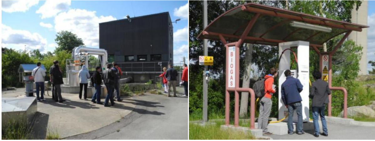
Picture 4: On the top of a digester at Henriksdal biogas plant (left), inspection of the company owned biogas filling station for cars from Stockholm Vatten (right)
