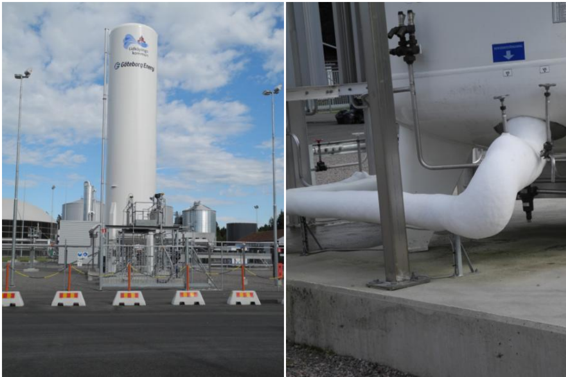
Picture 20: LBG storage tank (left) and frozen tube at the LBG storage tank (right)
