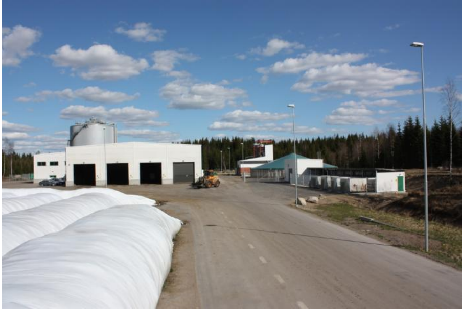
Picture 5: The Västerås biogas plant [picture: VafabMiljö]
