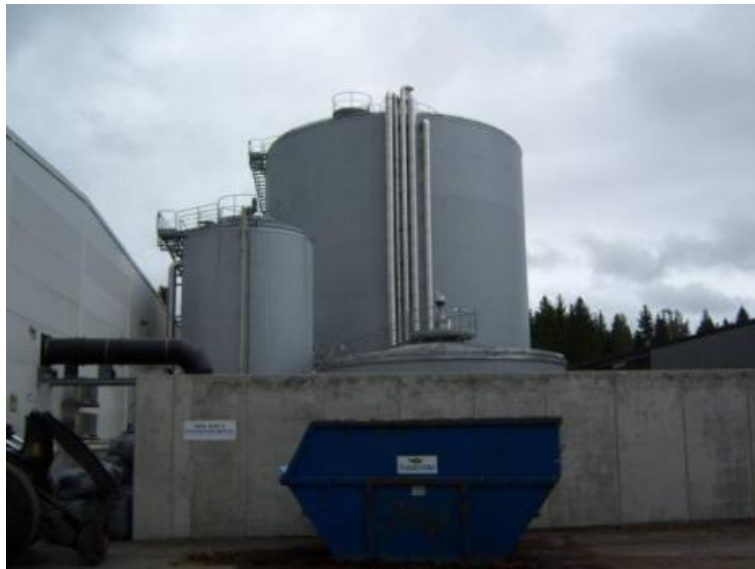
Picture 7: Digester and suspension buffer tank of the biogas plant
