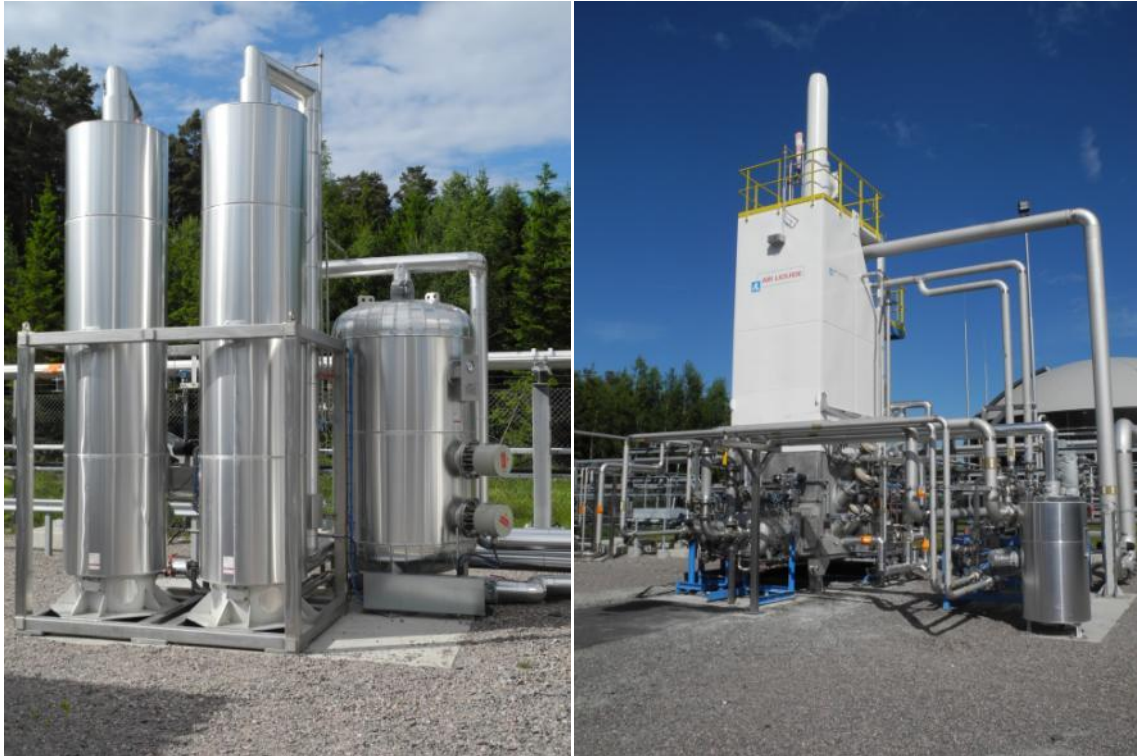
Picture 19: Pressure swing adsorption upgrading plant (2 nd upgrading plant) (left); LBG (Liquid BioGas) production plant (right)
