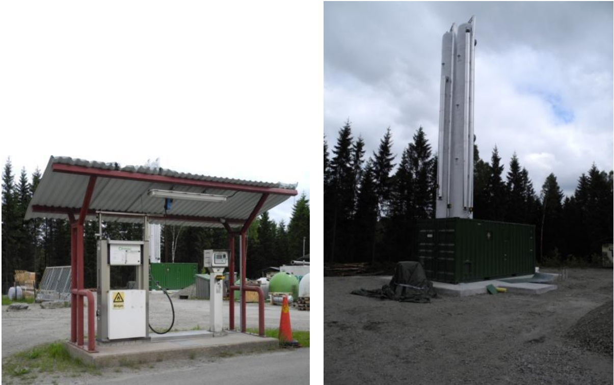
Picture 28: Company biogas filling station at the biogas plant site (left), new implemented water scrubber upgrading plant
