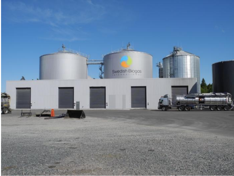
Picture 15: Biogas plant from Swedish Biogas international at Lidköping
