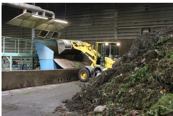
Figure 11: UrbanBiogas study tour: MSW reception hall of the Ganser biogas plant in Munich, Germany
