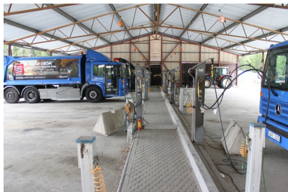
Figure 5: Long-term biomethane filling station for waste trucks in Sweden at the UrbanBiogas study tour
