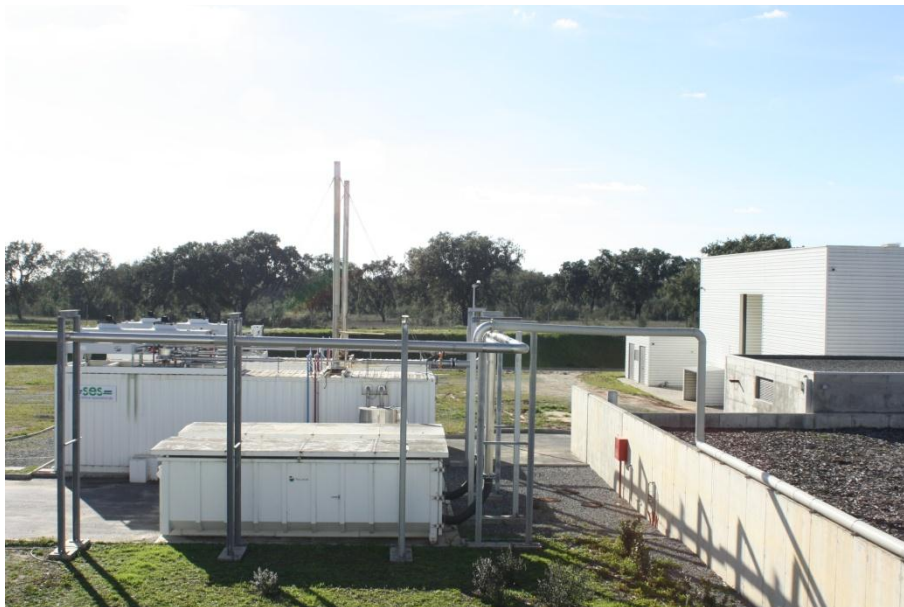
Figure 31: Visit to Valnor – unit of biogas
