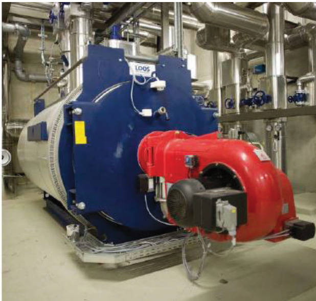
Picture 33 and 34: High temperature boiler with 1,7 MW and heat exchanger to district heating net (source: MA48 Stadt Wien)
