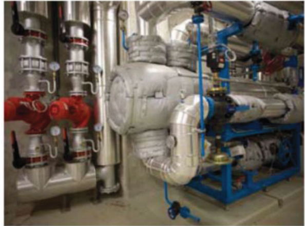
Picture 33 and 34: High temperature boiler with 1,7 MW and heat exchanger to district heating net (source: MA48 Stadt Wien)
