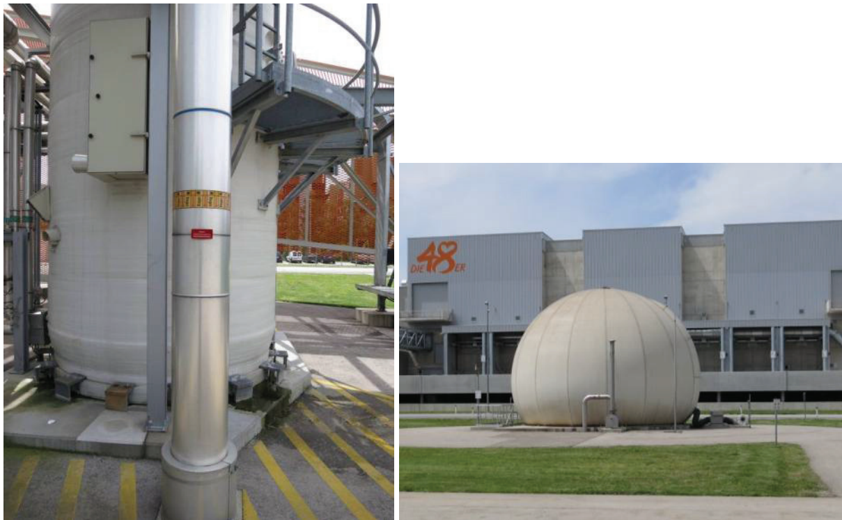
Picture 31 and 32: Desulphurisation and gas tank with 400 m 3 (source: GEA)
