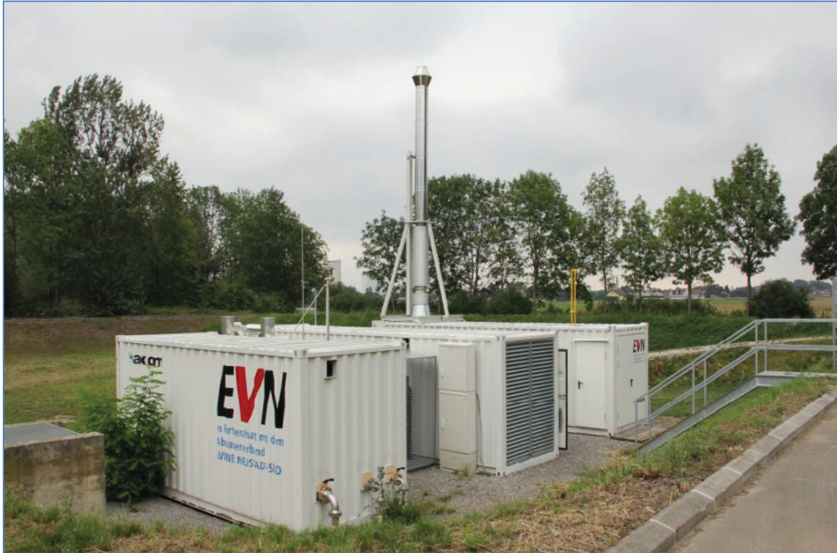
Picture 17: Biomethane plant Wiener Neustadt (source: EVN)
