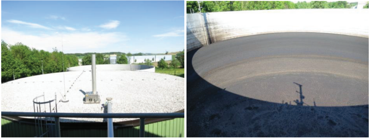
Picture 13 and 14: Secondary fermenter and residue storage tank (source: GEA)
