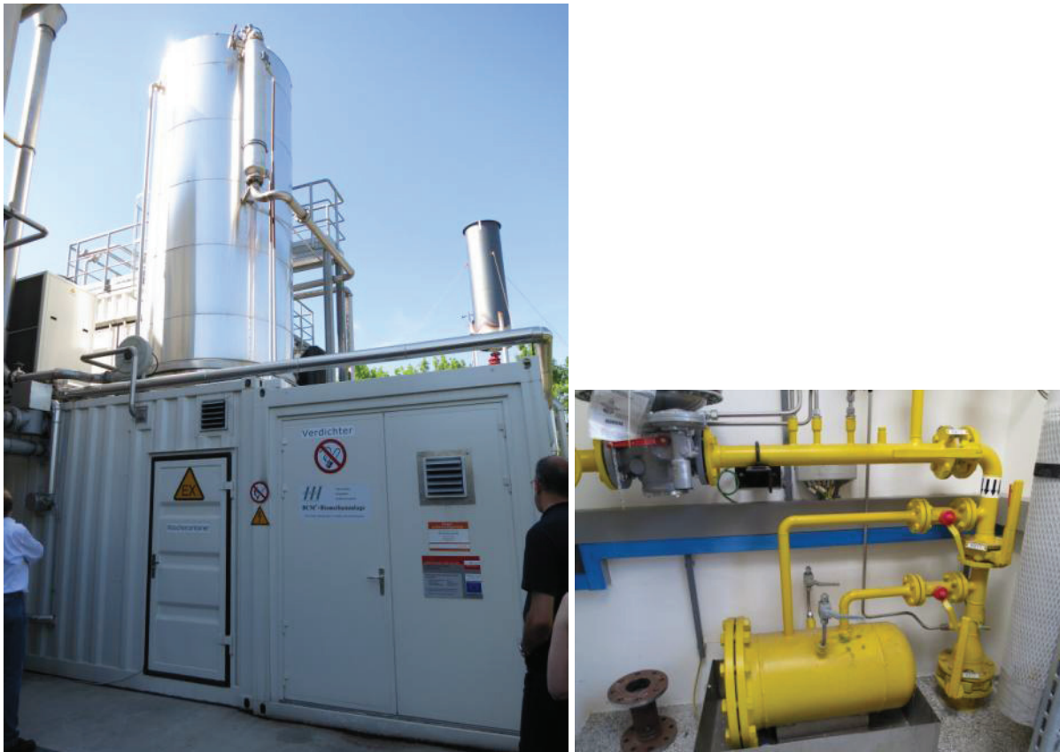
Picture 15 and 16: Amine-upgrading plant; addition of propane and odourisation (source: GEA)
