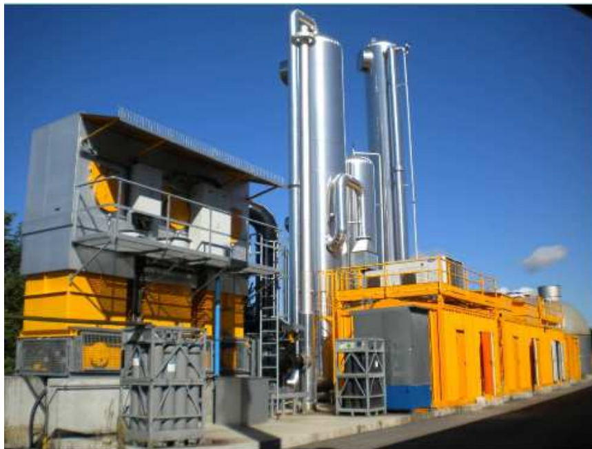
Figure 4-20 Water scrubber (with regeneration) upgrading unit (Fraunhofer, IEE UrbanBiogas, 2012)
