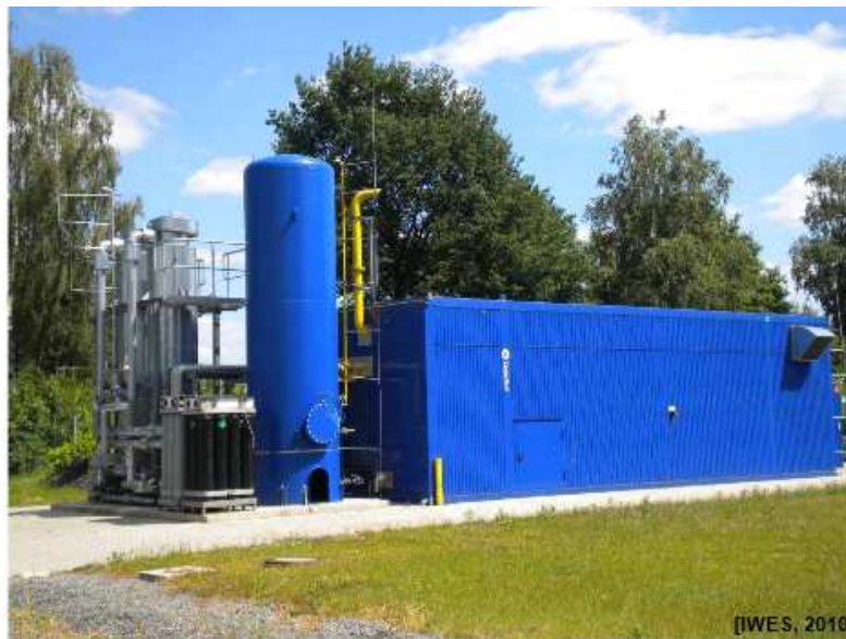
Figure 4-22 PSA upgrading unit (Fraunhofer, IEE UrbanBiogas, 2012)
