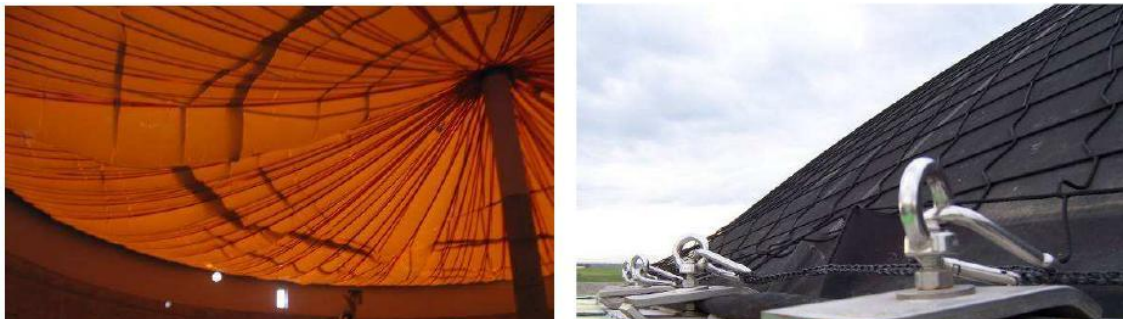
Figure 22 - Digester cover of gas tight membrane, seen from the inside of the tank - left (AGRINZ 2006); Digester cover of gas tight membrane, outfitted in exterior with expansion net - right (RUTZ 2006). (Source: Biogas Handbook)
