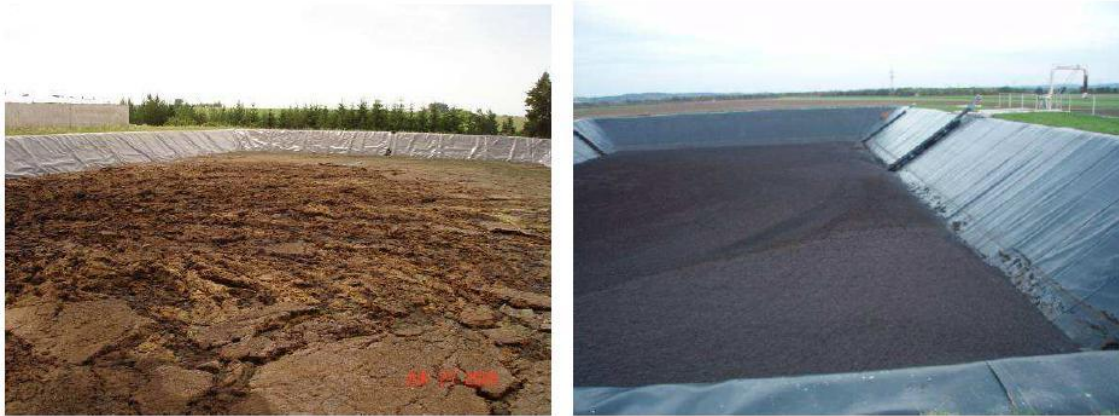
Figure 26 - Open pond lagoons for digestate storage (AGRINZ 2006). (Source: Biogas Handbook)
