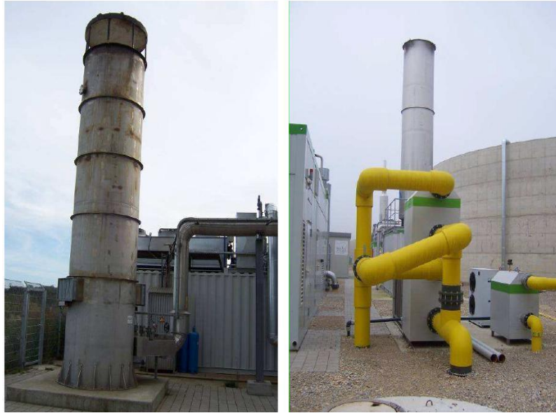
Figure 23 - Modern biogas flares (RUTZ 2007). (Source: Biogas Handbook)
