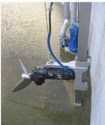
Figure 19 - Submersible motor propeller stirrer (AGRINZ 2006). (Source: Biogas Handbook)
