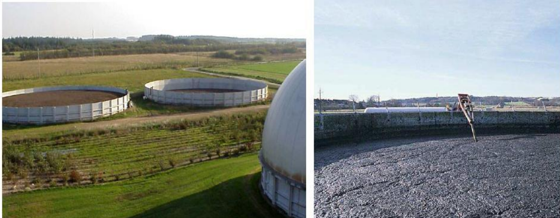
Figure 25 - Storage tanks covered with natural floating layer (DANISH BIOGAS ASSOCIATION 2008). (Source: Biogas Handbook)
