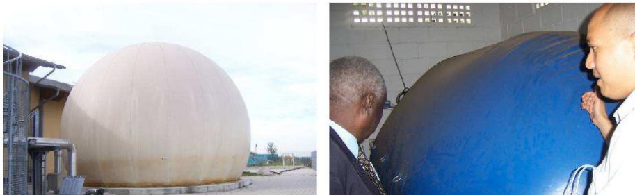
Figure 21 - External low pressure gas storage tanks (RUTZ 2007). (Source: Biogas Handbook)
