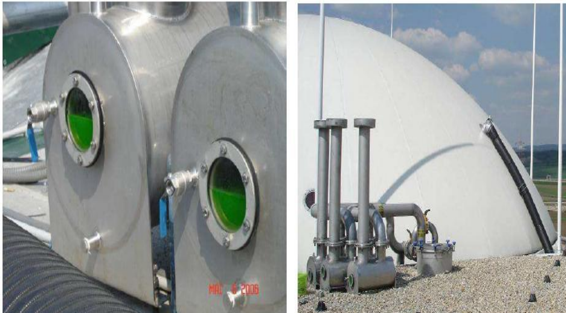
Figure 20 - Safety pressure facilities and valves (AGRINZ 2006). (Source: Biogas Handbook)
