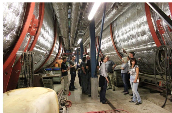
Figure 7: UrbanBiogas study tour: Digesters of the biogas plant for organic household waste of WurzerUmwelt in Eitting, Germany
